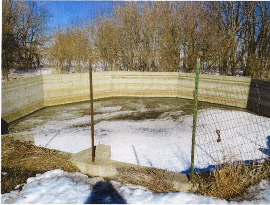
Manure storage – 40'd; 95,000 gal. capacity
