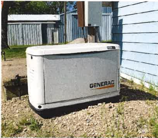
Standby generator – 20 Kwh
